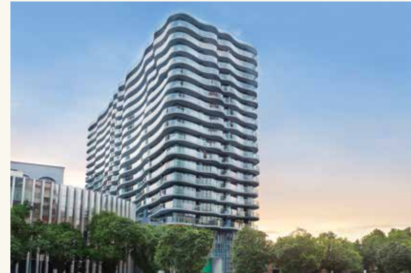
≈ 翠湖豪庭, 35 Albert Road, South Melbourne.
